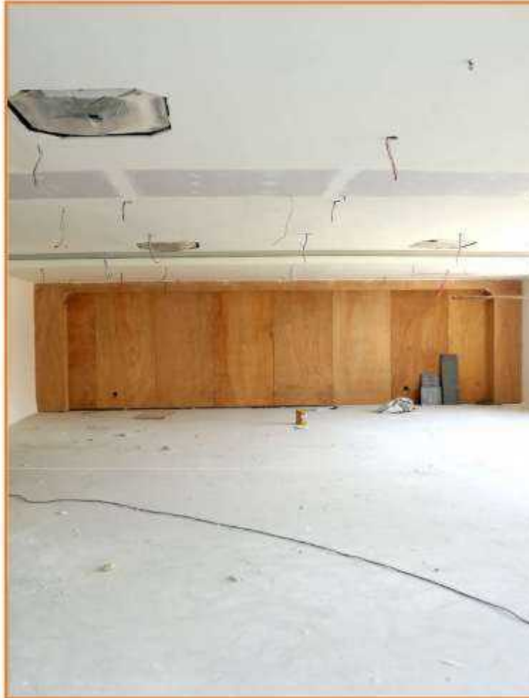
1st Floor - Activity Studios Gypsum Falseceiling & Wall Primer on 25/03/2025
