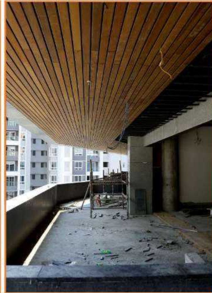
3rd Floor Wooden Ceiling work on 25/03/2025
